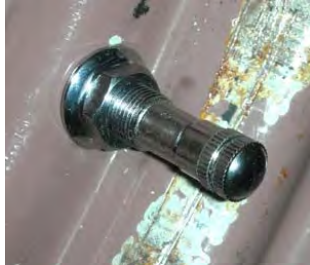
Metal stem installed
