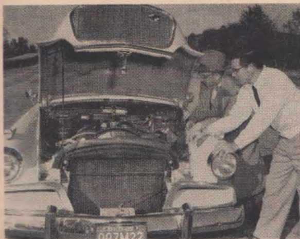
Studebaker Engineer Ed Reynolds gives Fermoye a briefing on the 352-cubic-inch engine. Note the novel hood-grille combination on this pre-production car.
